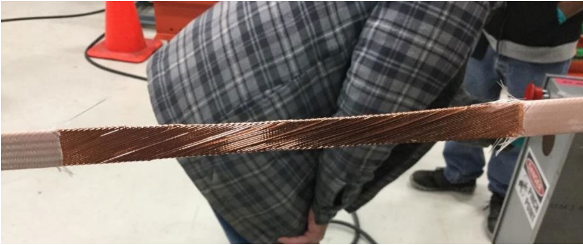
Figure 9.5: Coil 123 roped cable after insulation was removed, and before cable was fixed
