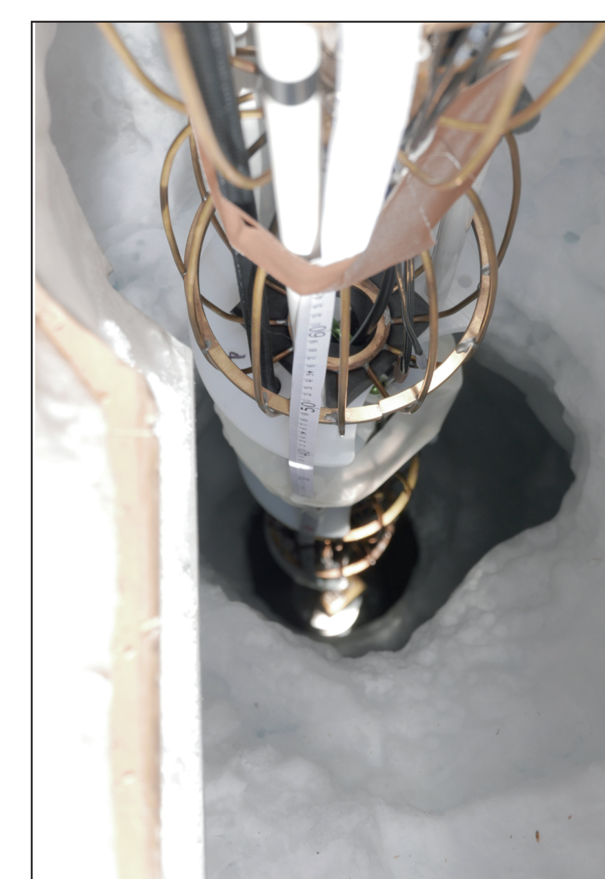
Left: ARA deployment down a borehole (E. Oberla).
